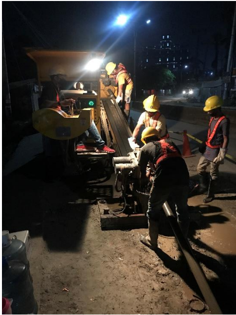
Picture 8 and 9: HDD work being carried out at nighttime on the roadside. SCL ensures that proper protective gears and jackets are worn all the time during work. Adequate lighting is provided for work and the workers to be visible for others. Night-time is the preferred time for HDD work in dense traffic areas as there is less possibility for traffic disturbance.
