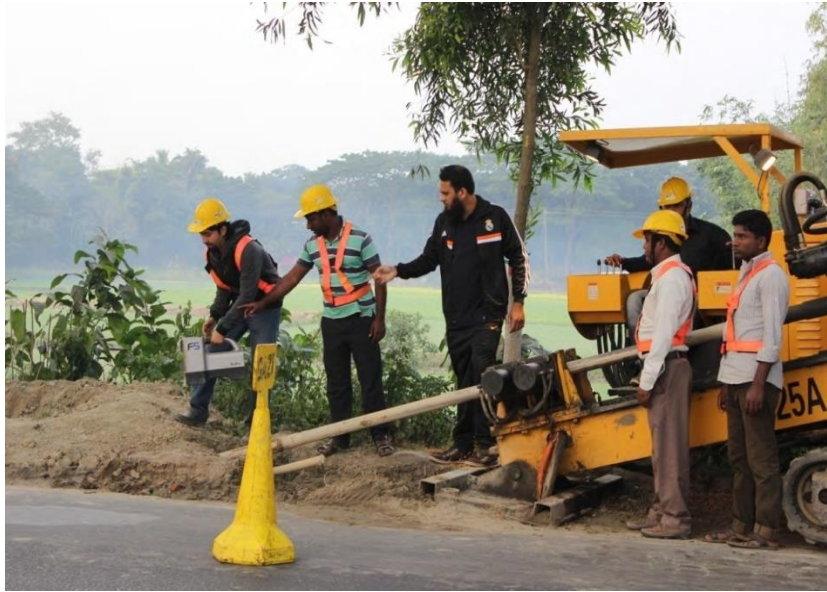
Figure 3. 6: Horizontal Directional Drilling (HDD) Machine
