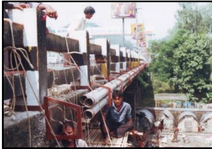
Figure 3.10: Bridge crossing of fiber optic cable using DWCP Pipe with Clamping.
