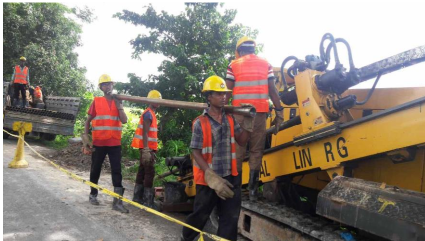
Picture 2: Workers wearing safety gears and PPE and conducting HDD operation during daytime at the roadside
