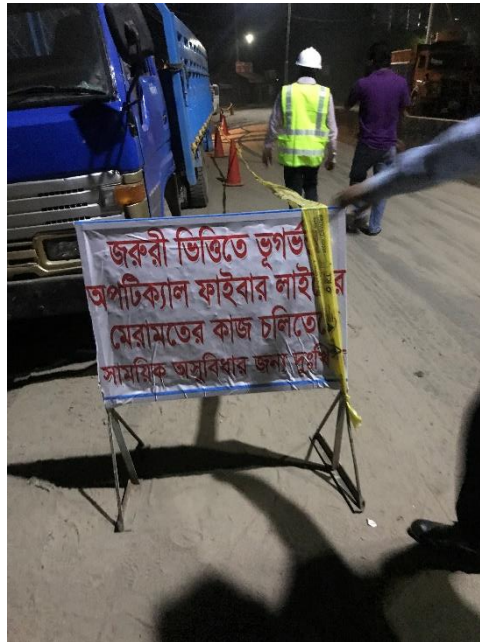
Picture 7: HDD work going on during night-time at roadside. SCL ensures that the precautionary signs and tapes are visible at dark by providing adequate lighting.
